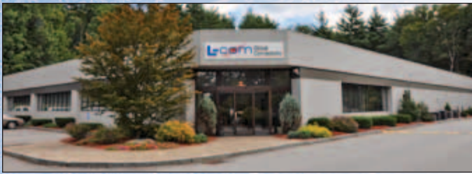
L-com's Corporate Headquarters & Fulfillment Facility, North Andover, MA 01845, USA
