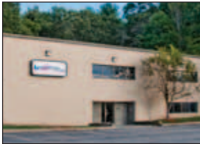
Cable Assembly Manufacturing Facility, North Andover, MA 01845, USA
